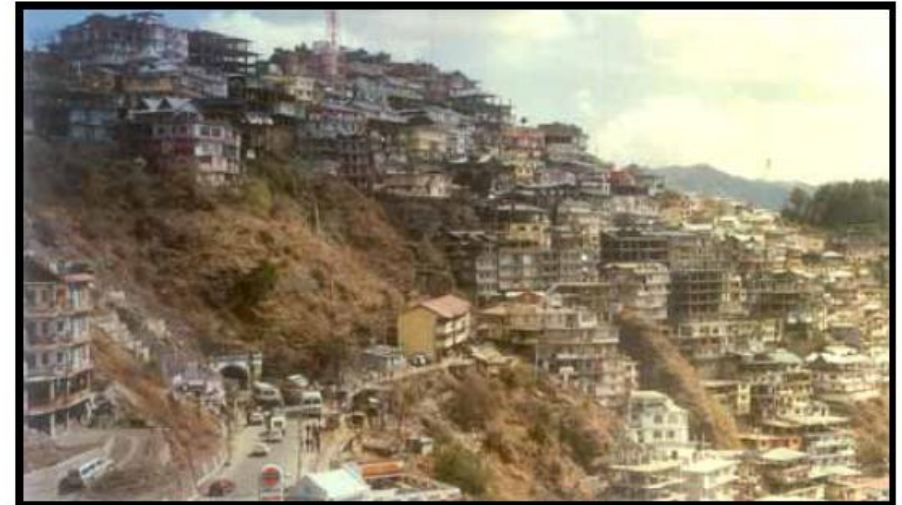
Massive Construction at Cemetery without Proper Accesses
